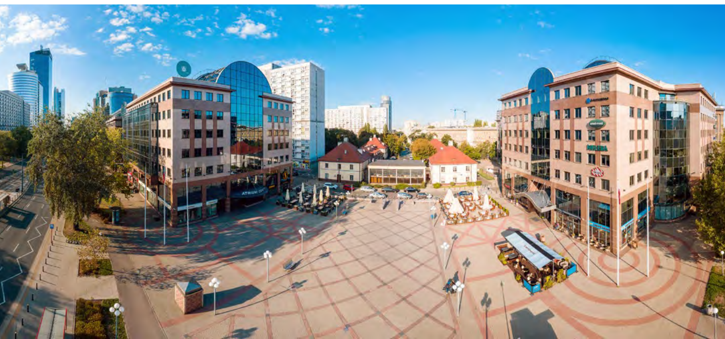
Atrium Complex, Warsaw, Poland
