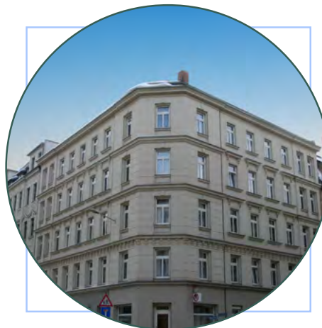
Residential Apartments, Leipzig, Germany
